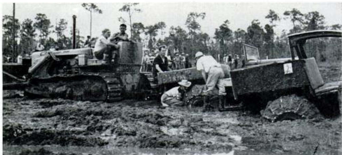
Mired swamp buggies keep the rescue bulldozer busy. Axles of these racers are submerged in sticky goo
